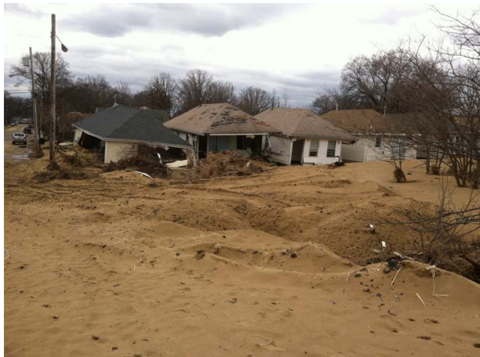
Figure 8. Homes with damage from Hurricane Sandy
