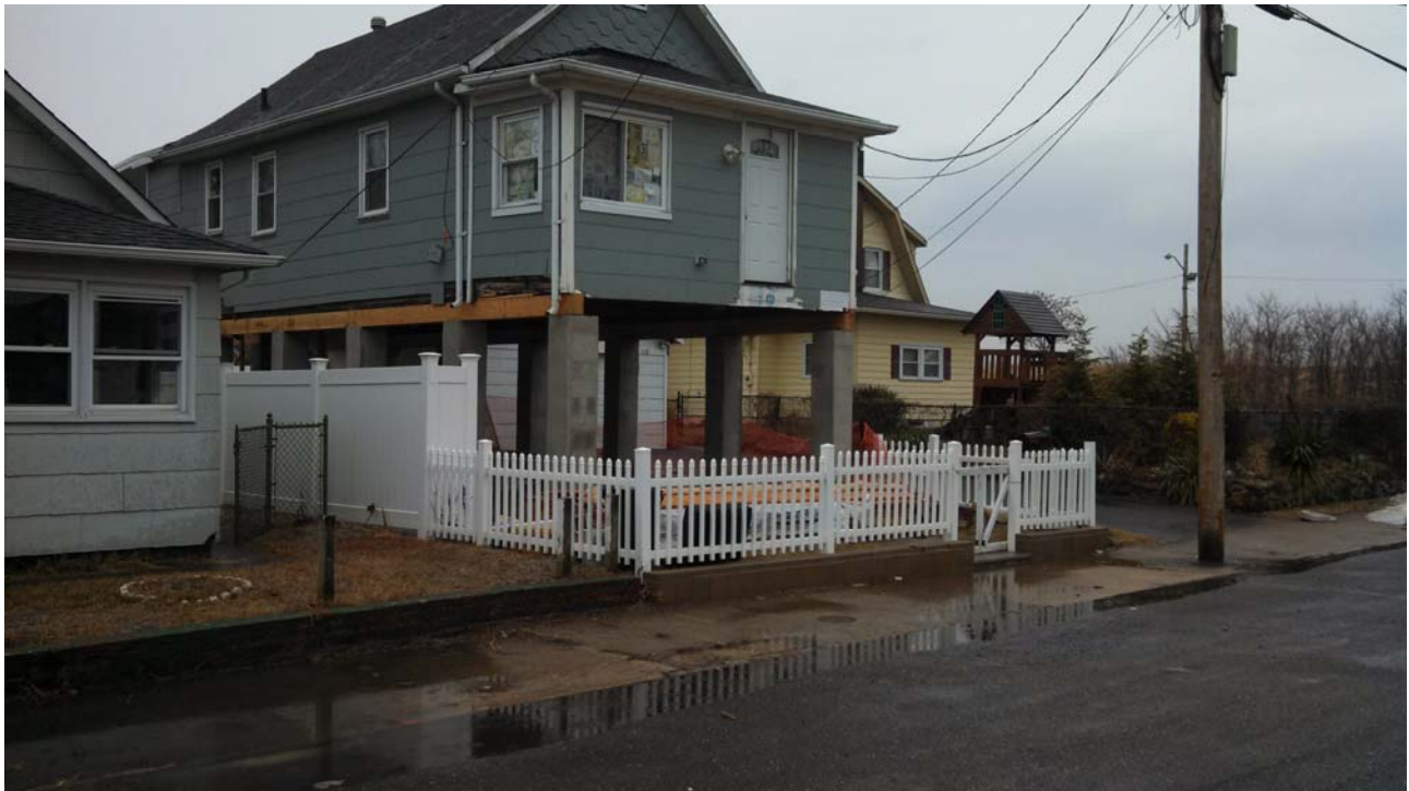
Figure 10. Existing home elevated to meet BFE standards in Keansburg
