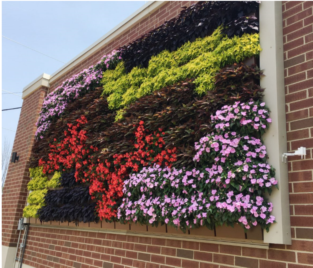
Example of live wall (Source: www.livewall.com )
