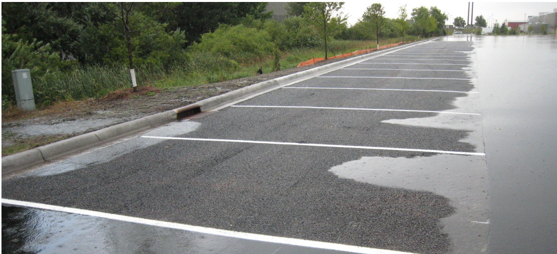
Example of permeable pavement (Source: Potomac Conservancy)
