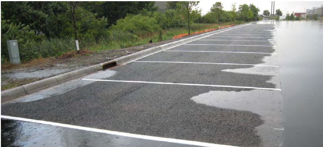
Example of permeable pavement (Source: Potomac Conservancy)
