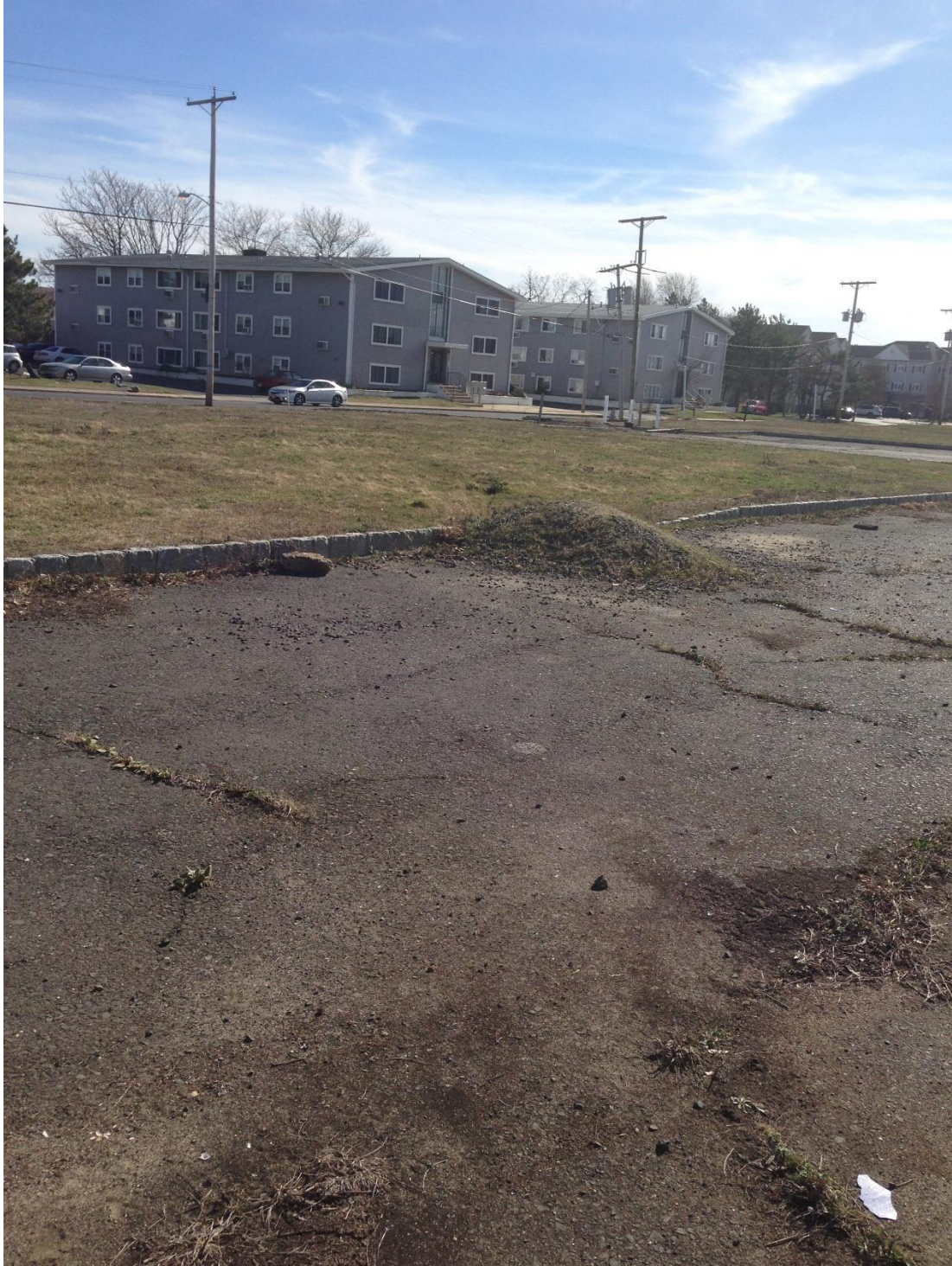
Picture 5: View from Ex. Parking Area Ave Looking South
