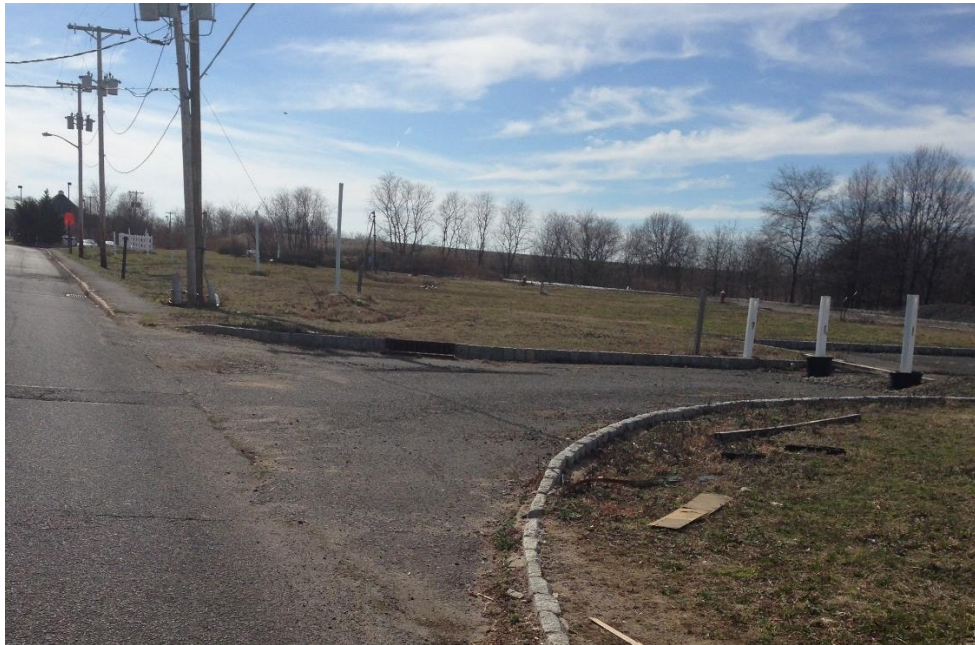
Picture 2: Beachway Avenue Looking West
