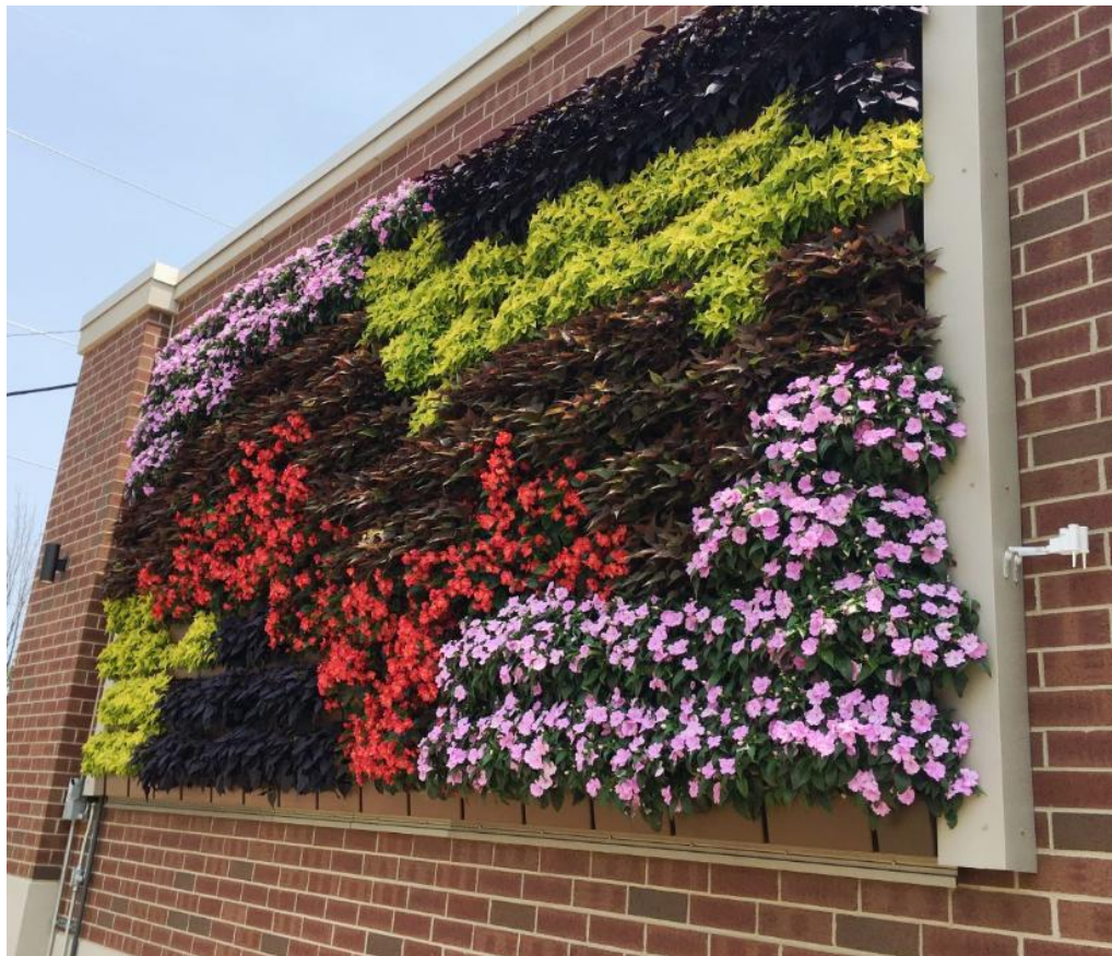
Example of live wall (Source: www.livewall.com )
