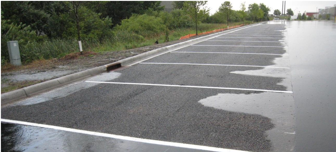
Example of permeable pavement (Source: Potomac Conservancy)
