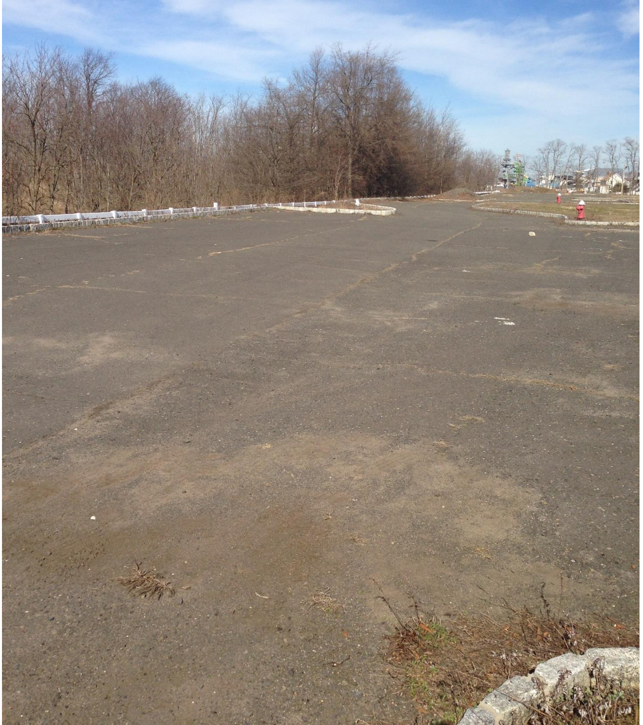
Picture 4: Ex. Parking Area Looking Northeast
