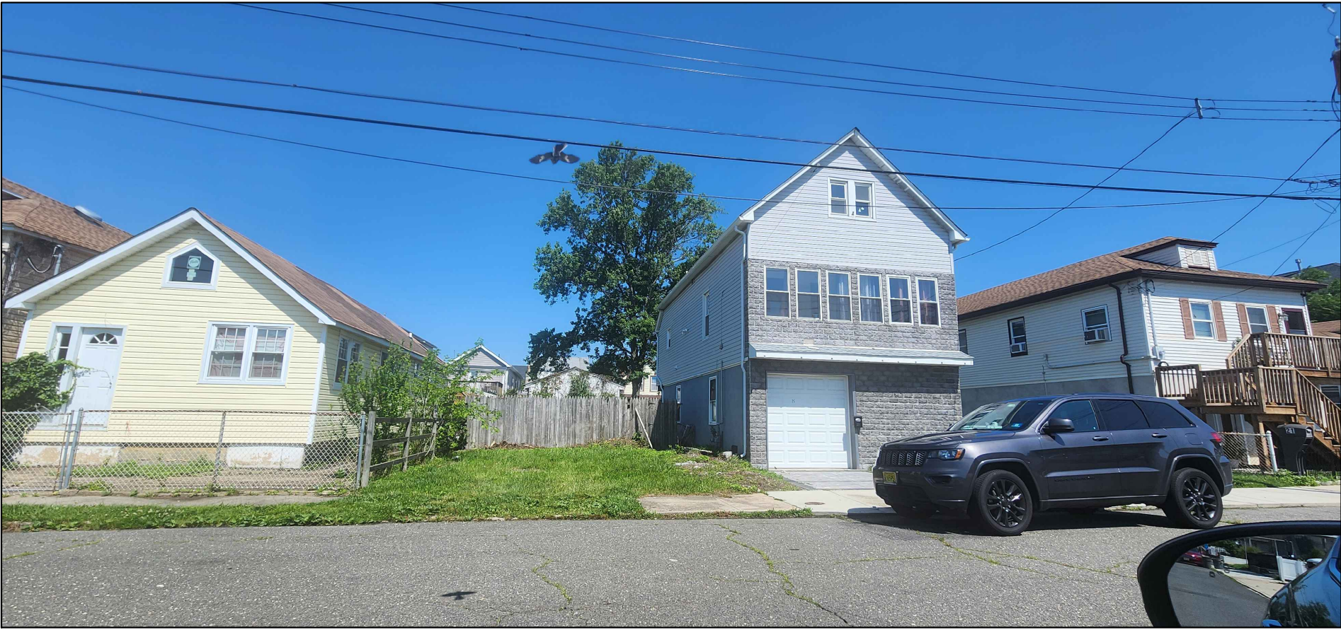
VIEW OF EXISTING LOT
